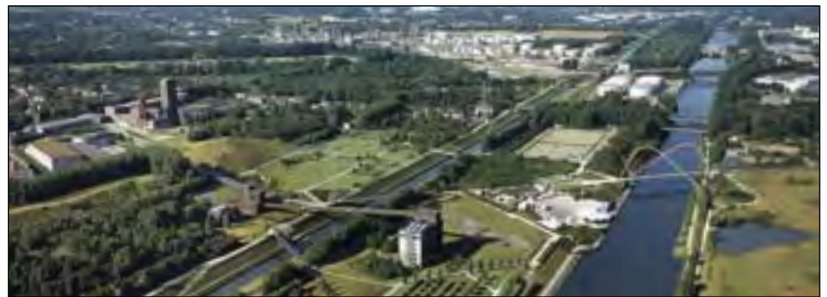
1.1.5 Emscher zone: Landscape of bridges in the Gelsenkirchen Nordstern Park with the Emscher island and the open-air theatre
