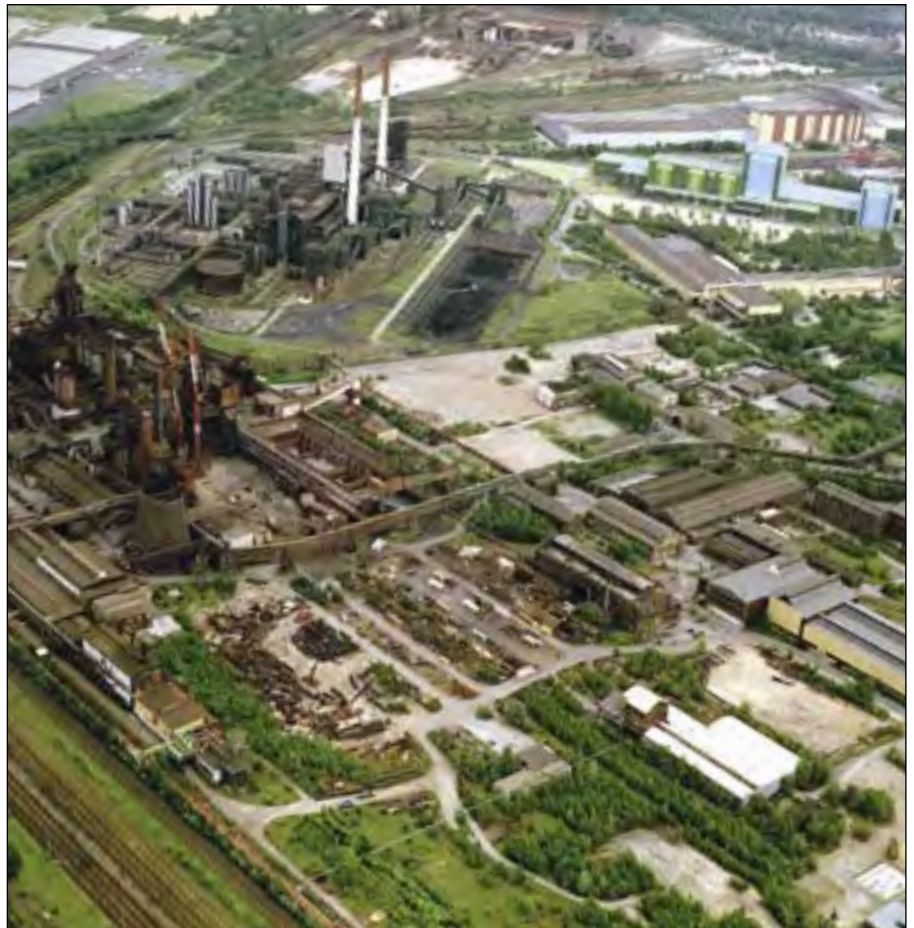
3.1.9 Smelting plant Westfalenhütte in Dortmund in 2002, being dismantled to be transported to China
