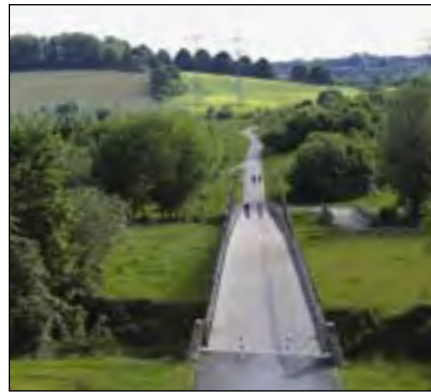
1.1.3 A Hellweg zone green belt: The Mechtenberg bridge in Gelsenkirchen
