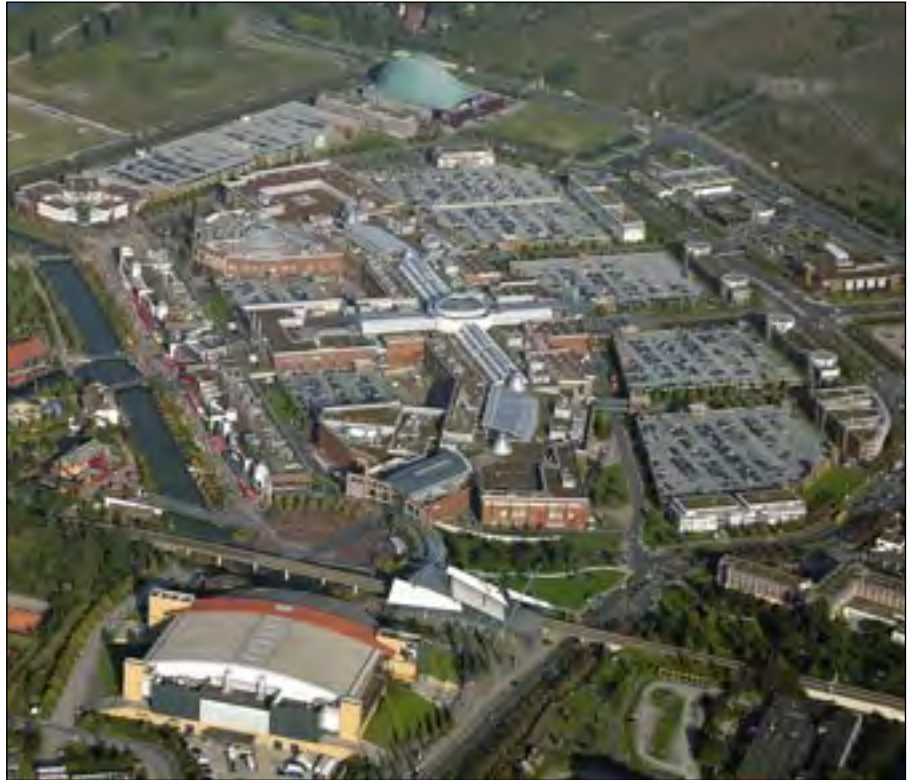
3.5.1 Neue Mitte Oberhausen (CentrO shopping center in the middle)
