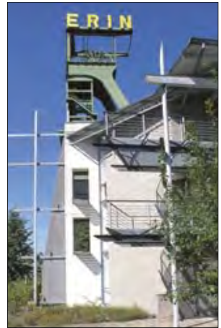
4.3.12 Industrial and office park on the site of the former Erin mine in Castrop-Rauxel
