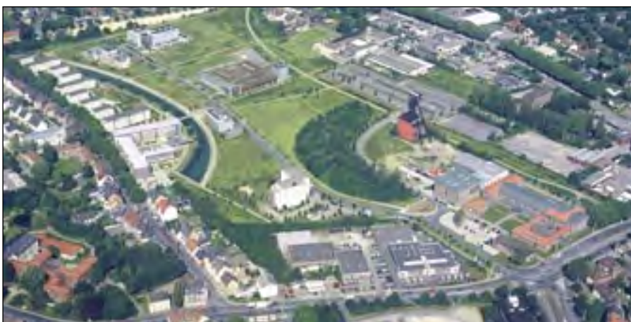
2.4.9 Housing quarter and industrial park on the Holland mine site in Bochum-Wattenscheid
