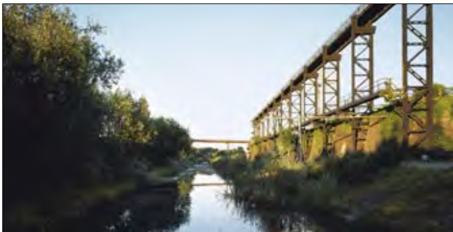
1.2.11 The renaturated Alte Emscher in the Landscape Park Duisburg North
