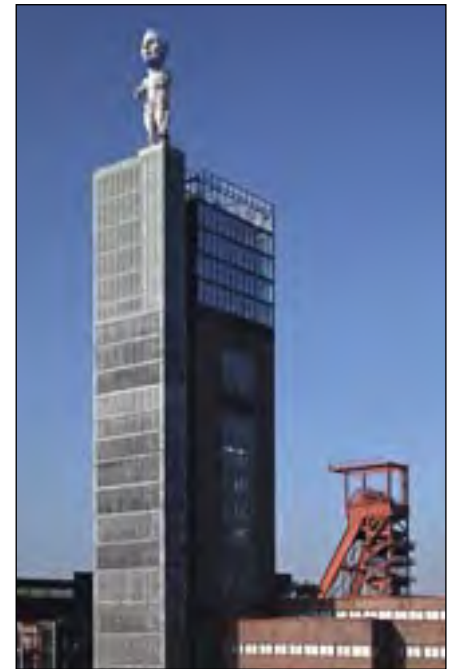
2.5.1 Hercules sculpture on the extended winding tower of the Nordstern mine in Gelsenkirchen
