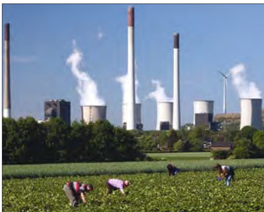
3.3.4 Coal power station in Gelsenkirchen-Scholven
