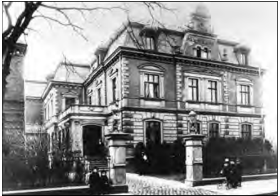
2.1.4 Old Amtshaus/City Hall in Herten (1892 to 1957)
