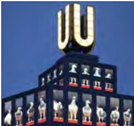
4.4.8 Dortmund U: once a cooling tower of the Union Brewery, now a center of culture with a video installation
