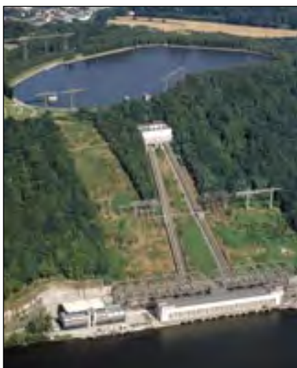
3.2.6 Pumped storage hydro power station "Koepchenwerk" on Lake Hengstey in Herdecke
