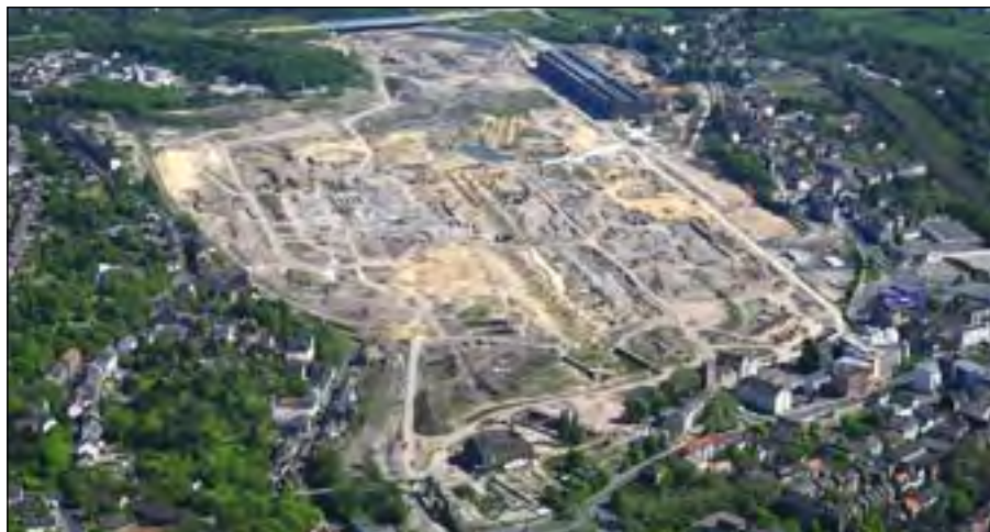
2.4.13 From the dismantled steel works Phoenix-East ...
