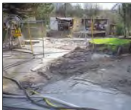
4.3.2 Damage caused by subsidence in Bochum
