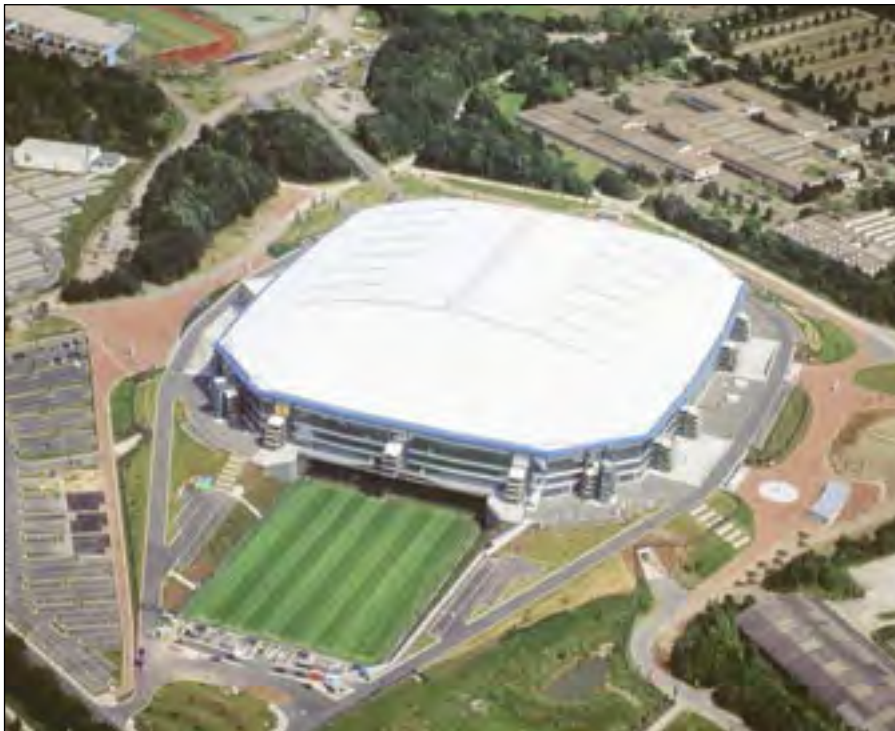
3.6.3 Arena AufSchalke in Gelsenkirchen, with the "lawn drawer" moved out and the roof closed
