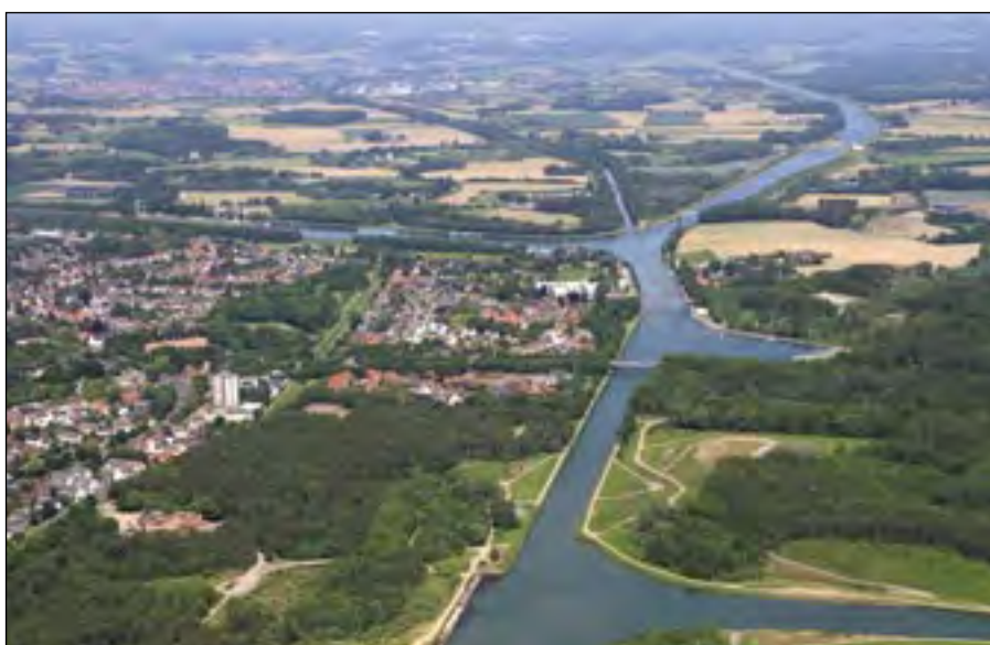
4.1.20 Waterway hub Datteln: Dortmund-Ems Canal (bottom), Datteln-Hamm Canal (to the right), Wesel-Datteln Canal (to the left) old and new speed of the Dortmund-Ems Canal (top)
